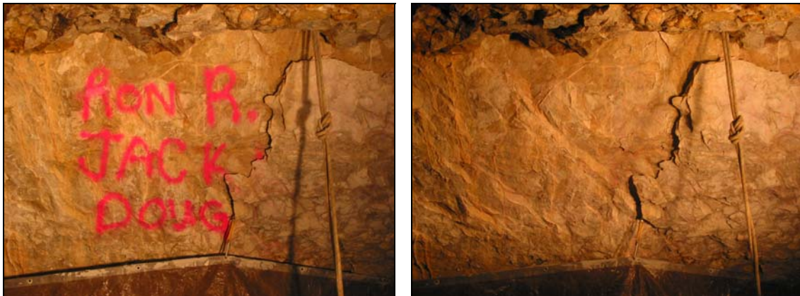
Before and after photo of graffiti being removed.
