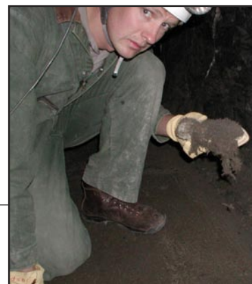
Lint and hair being removed from tunnel
