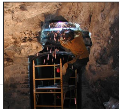
Installing a new cave gate
